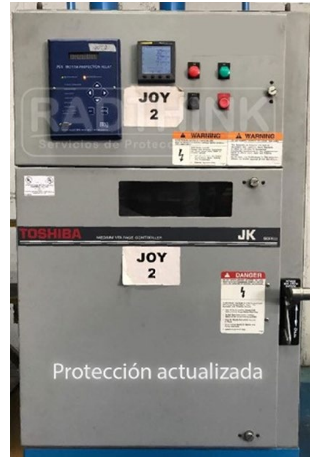
Fig. 2 Updated motor protection scheme.
