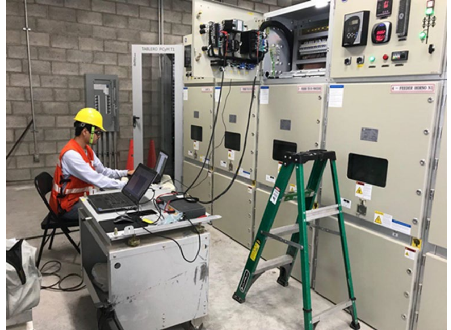
Fig. 2 Tests to protection relays.
