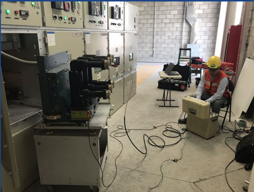
Fig.1 Hi-Pot tests to a medium voltage circuit breaker.
