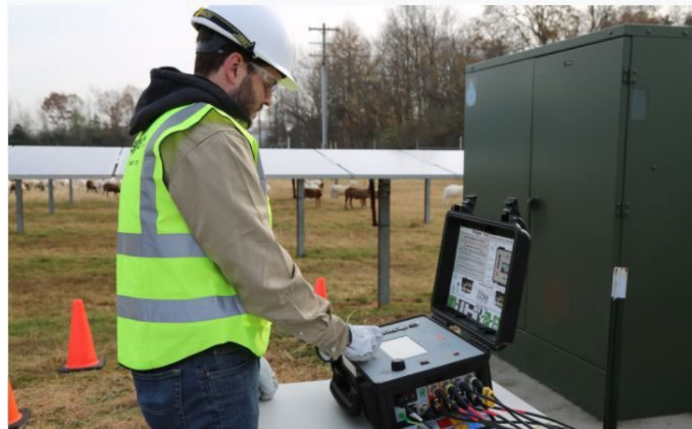
Fig. 2 Maintenance test of instrument transformers.
