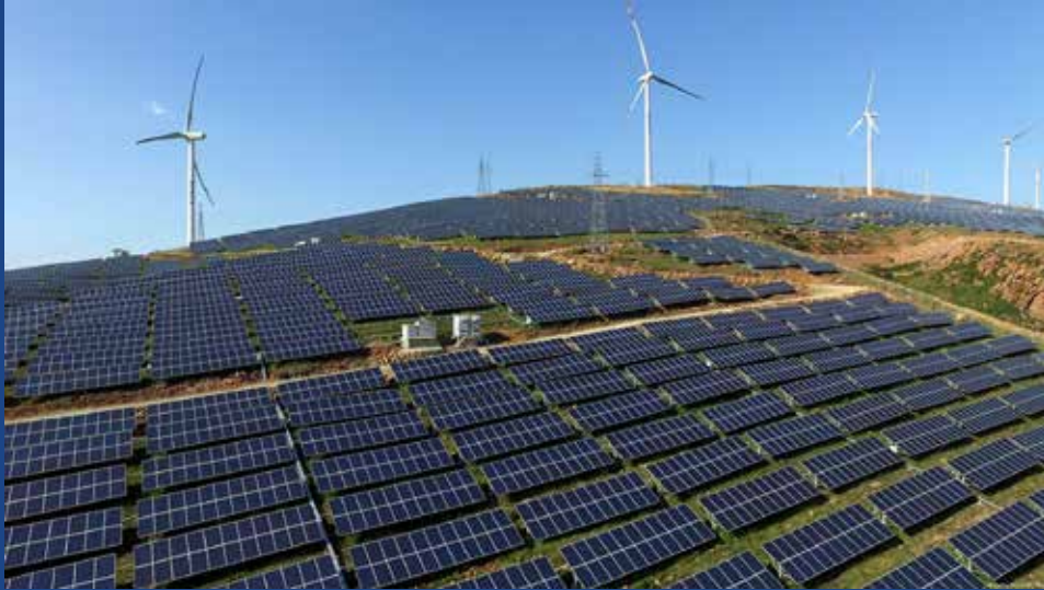
Fig. 1 Renewable Generation Plant
